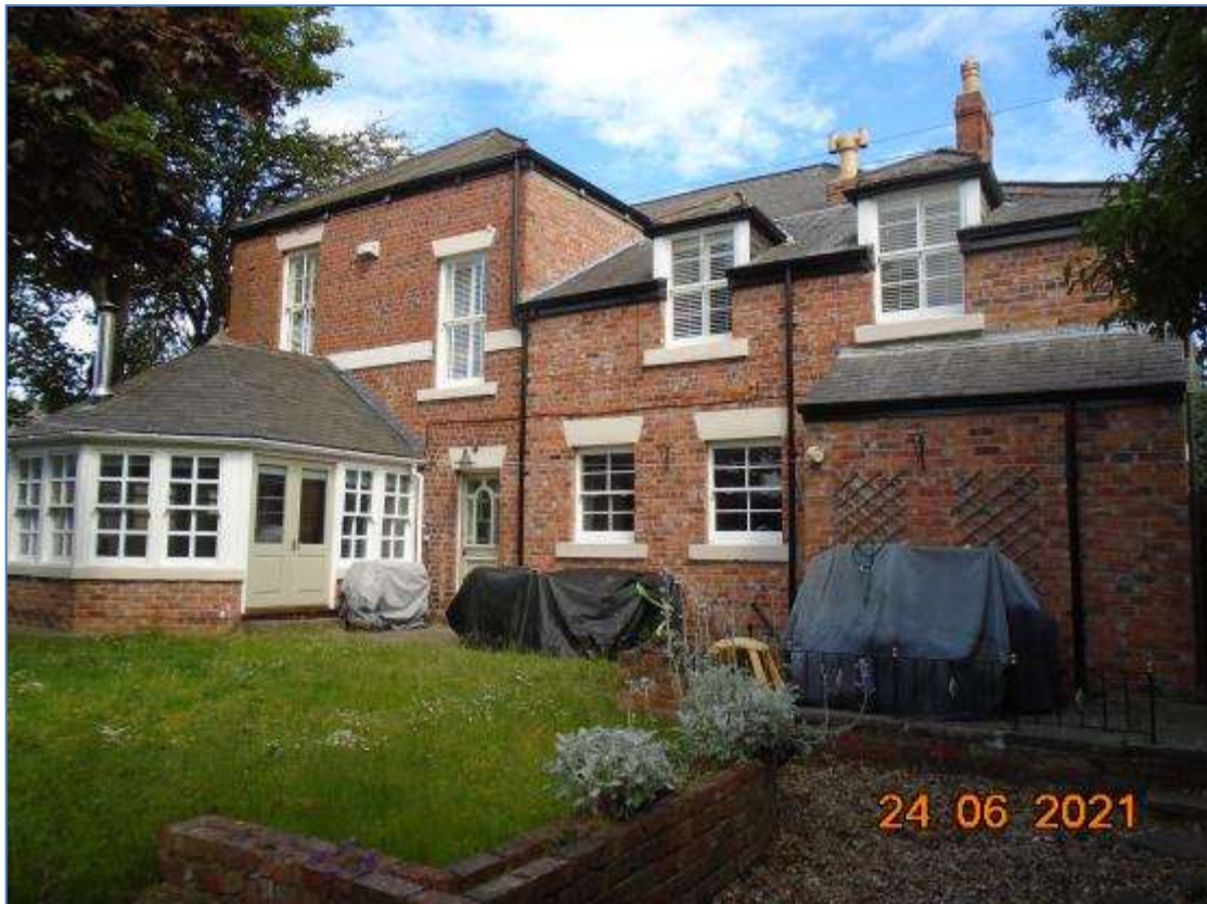
Photograph 2 – Rear (south) elevation of the property.
