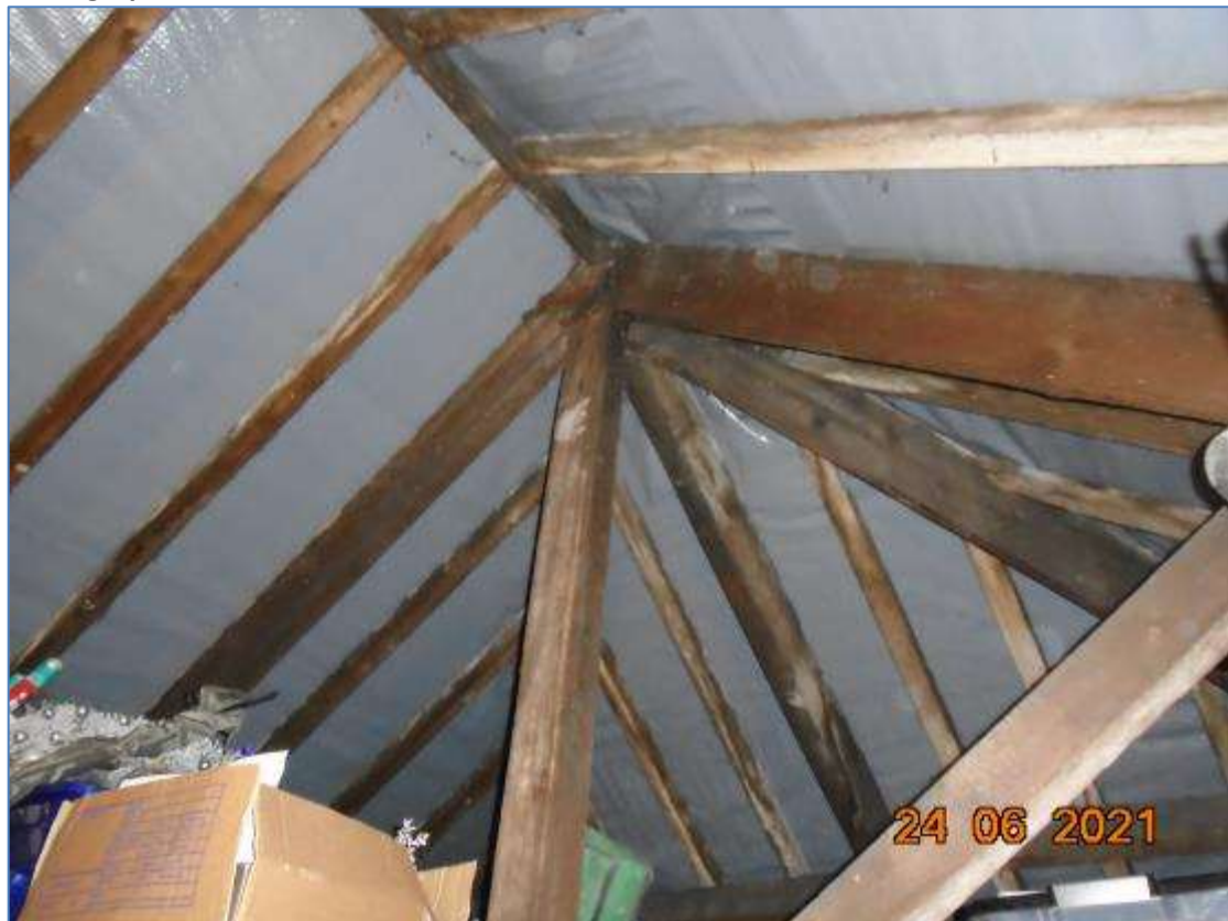
Photograph 6 – Internal view of the main roof structure.
